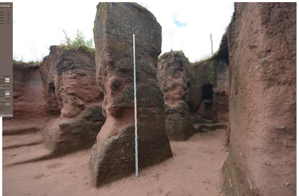
Beta Marqorewos, church on the site of Lalibela. Remains of pillars supporting a completely collapsed rock-cut arch. © mission Lalibela, 2016.
